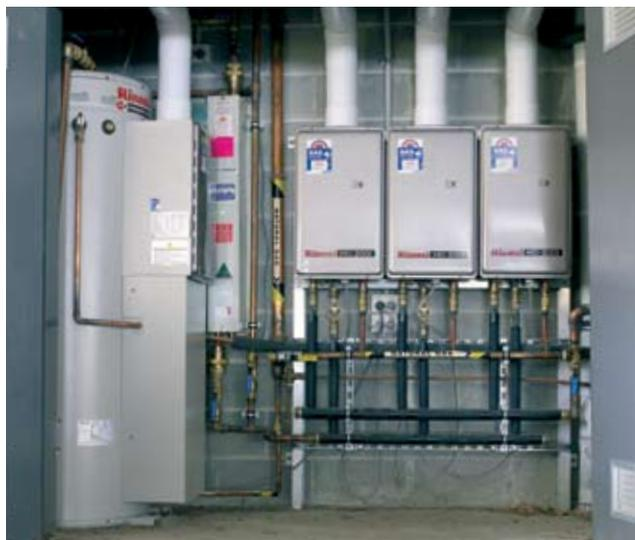
DD1 and Manifold Pack 3 with horizontal flueing. Note: now available with new front casing
