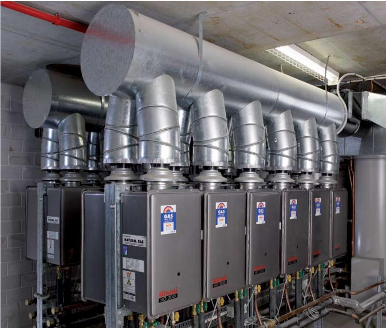
4 x DD6 back to back with 2 x Common Flue headers (power flue assisted)
