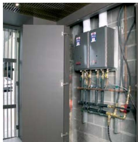
Manifold Pack 2 Internal installed in a cupboard
