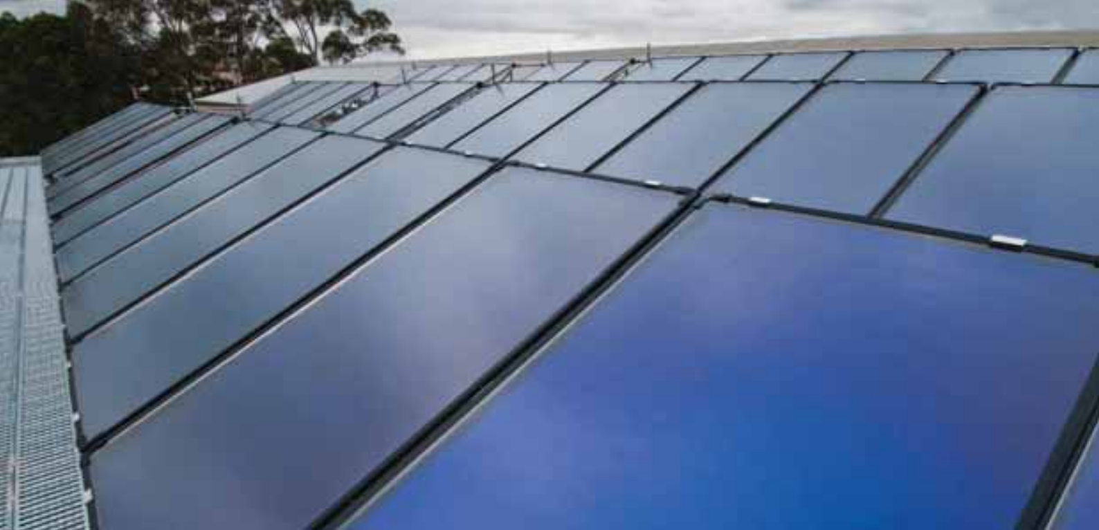
BT collectors at Rheem Testing Facility – Rydalmere – Australia
